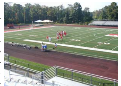
The track (shown above) was removed and re-installed.
