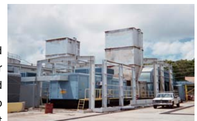
Partial Steel Framing, Gas Turbine at Dagua, Puerto Rico
