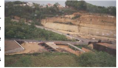
PR-115, Guayabo River Bridge, Aguada, Puerto Rico, looking east
