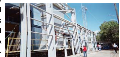
Partial Steel Framing, Gas Turbine Generators at Vega Baja, Puerto Rico
